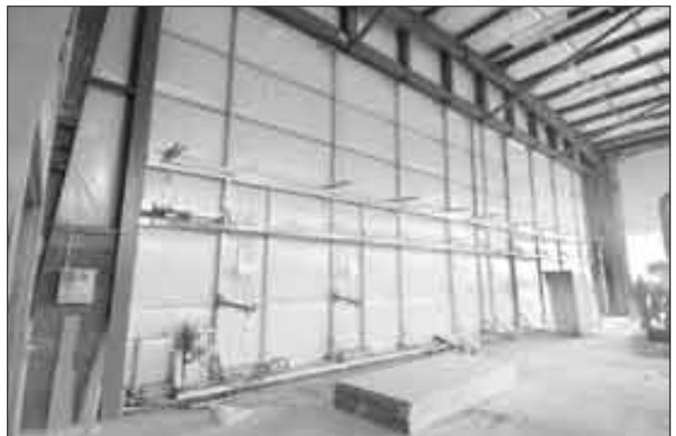
Helicopter access to the hangar will be through a 60- by 20-foot clamshell, aluminum door.
