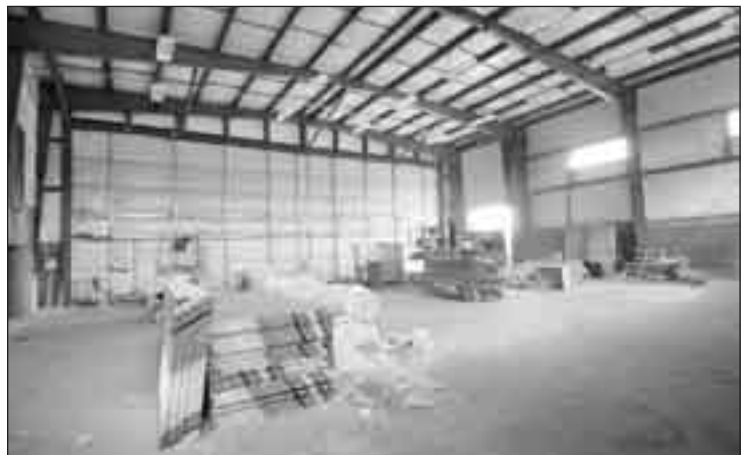
The 4,200-square-foot hangar with a 26-foot high roof will be used for maintenance and repair work on Winco's four helicopters.
