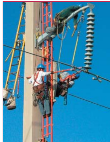
The new bells are moved into position and ready for installation.
